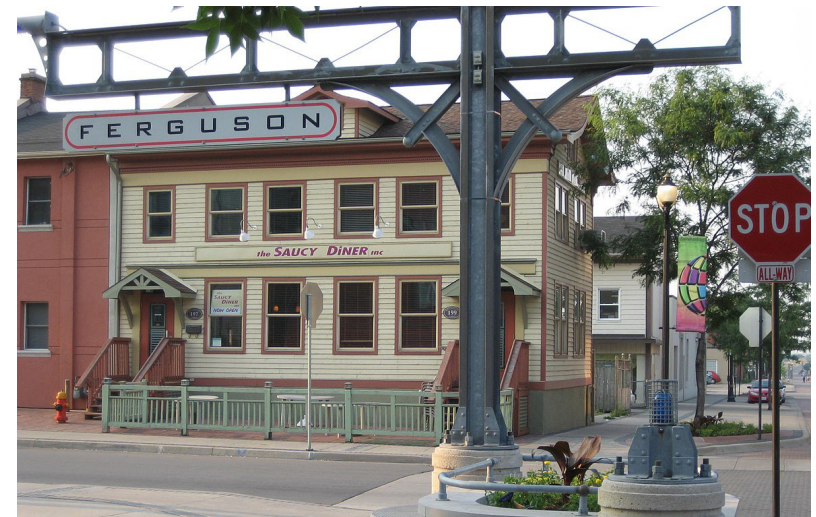
Fig 10. Ferguson Avenue Crossing Gates
