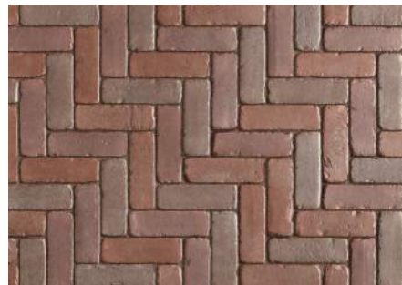
UPGRADED PAVING TREATMENT TO COMPLIMENT BUILDING FACADE IN HERRINGBONE AND STACKED PATTERN
