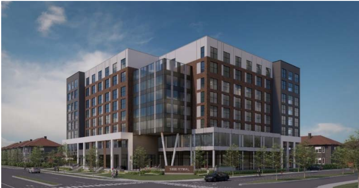
Figure 12- Rendering of Proposed Building from the Corner of Rymal Rd and Dakota Blvd.
